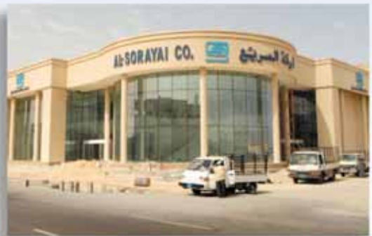
AL SORAYAI SHOWROOM, DAMMAM
